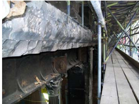
Existing cornice prior to preparation to receive new stonework
