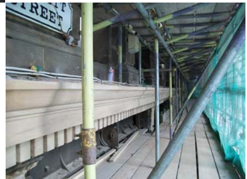
Stone cornice/dentils fixed back to existing structure
